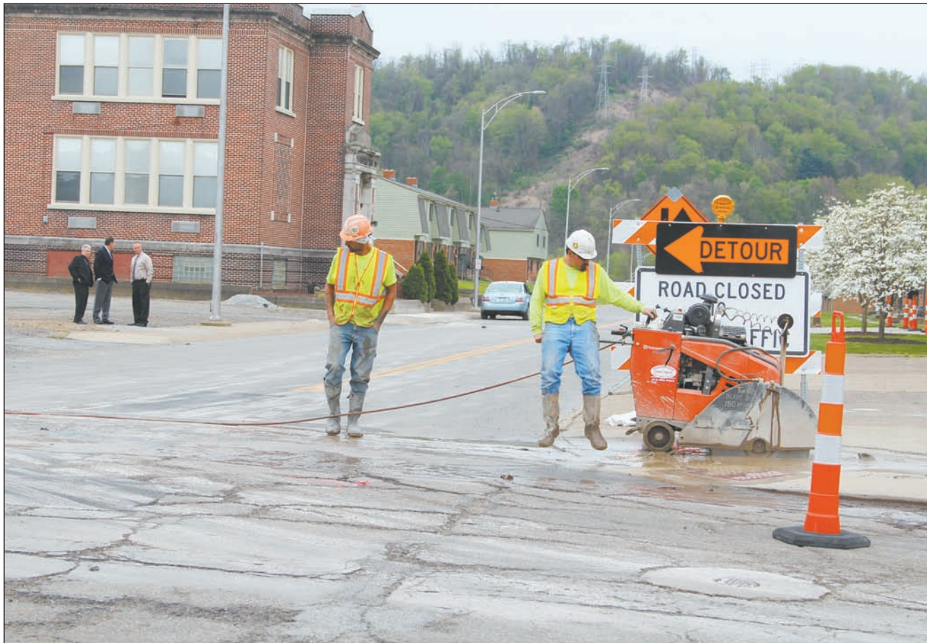
Workers from Concrete Coring Co., Butler, Pennsylvania, cut pavement around Holy Name Cathedral in preparation for installation of a cul-de-sac and pedestrian-friendly walkway. In the background, Diocese of Steubenville Bishop Jeffrey M. Monforton, his executive assistant, James G. Piazza, and D. Scott Yarman, project manager on the cathedral project, survey the work. (Photo by DeFrancis)
